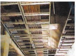
吊架 Tank Bridge
