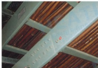
桥架 Bridge trestle
